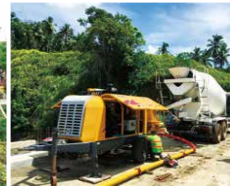
HBT8016V 江苏徐州 HBT8016V trailer-mounted concrete pump in Xuzhou, Jiangsu
